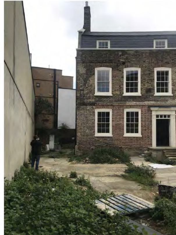
External - Rear (West)
